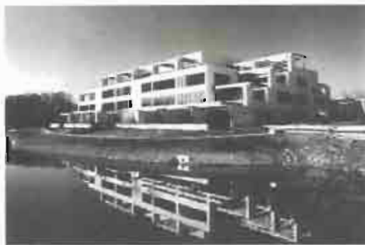
View from North-East
