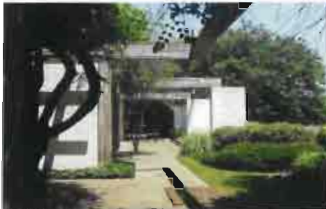
East Facade, with Lake Level Terrace
