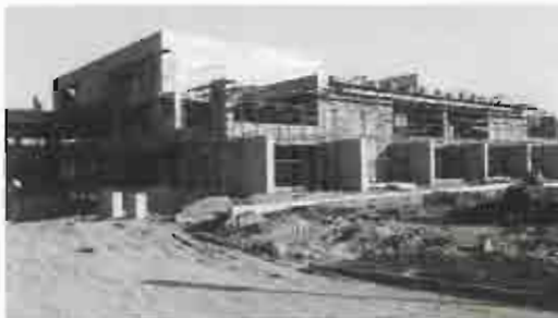
Concrete masonry unit solid walls
