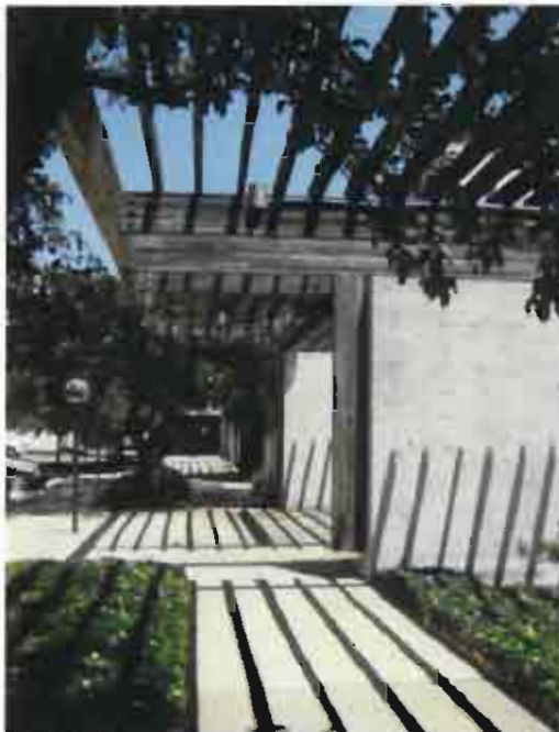
Wood Trellis at West Facade
