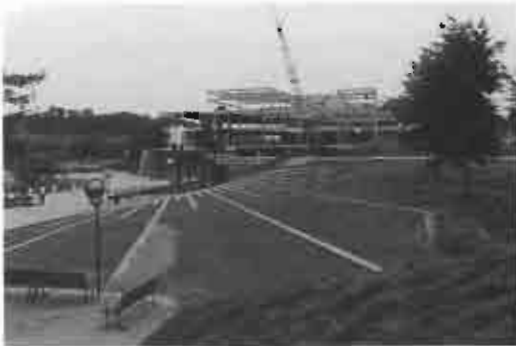
Steel framed building structure, under construction
