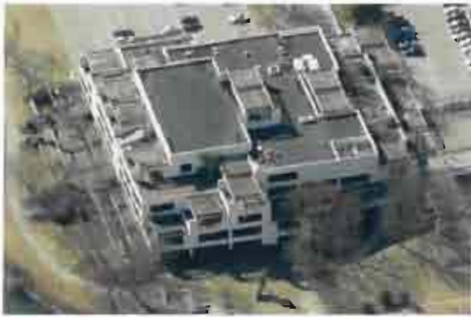
Overhead view from North-East
