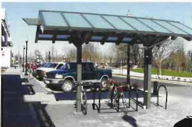
Covered Shelter Bicycle Parking Source: TDG Library
